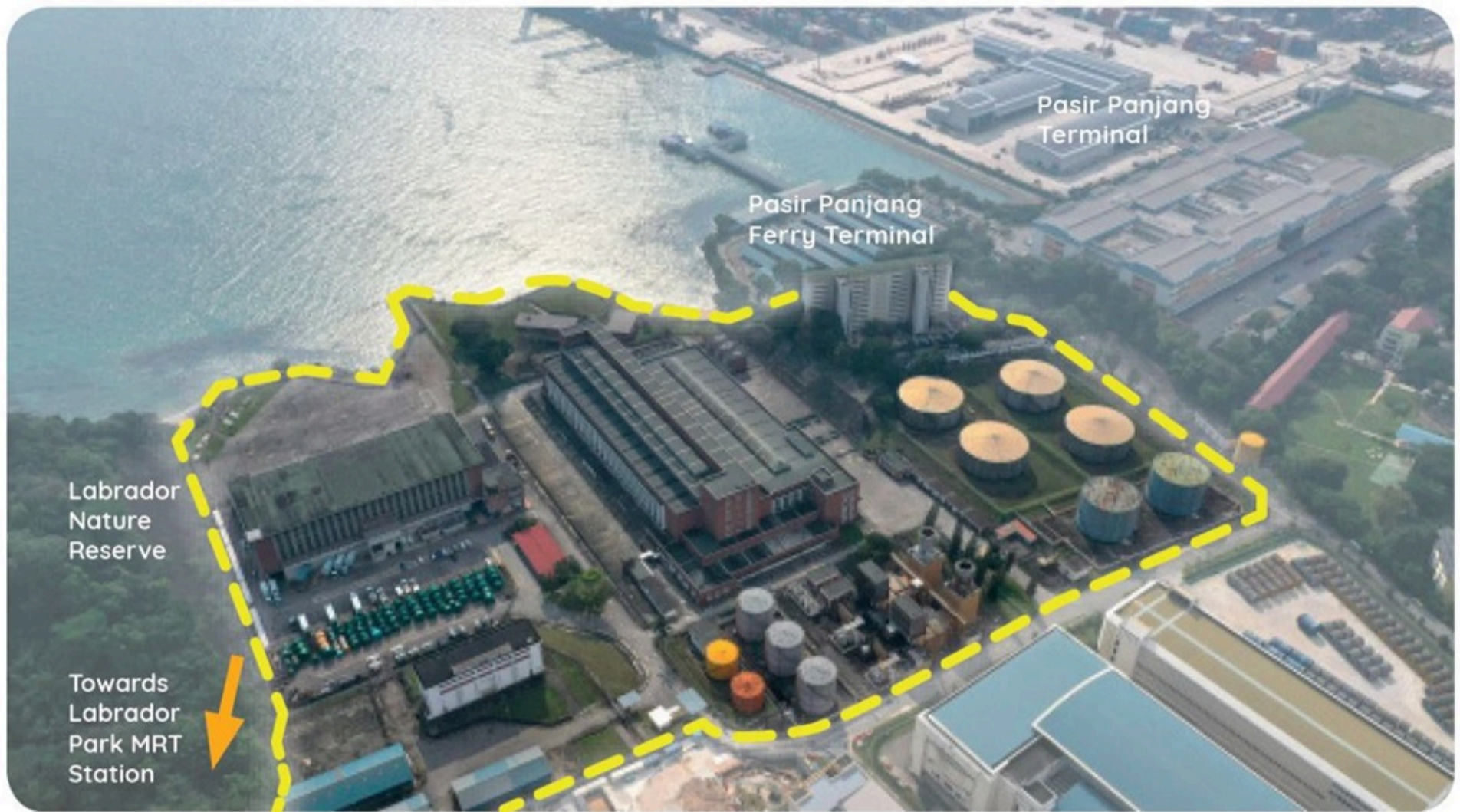
Aerial View of Pasir Panjang Power District
